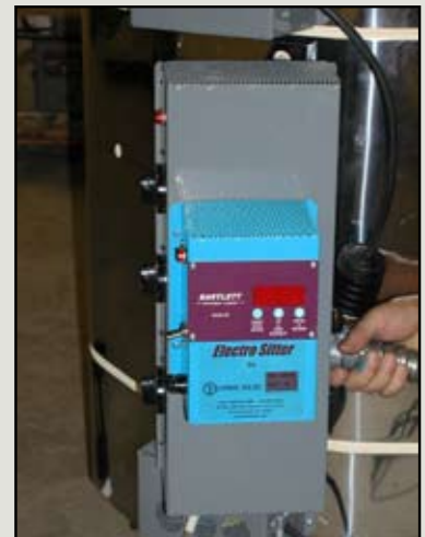
Install electrical box back on kiln with Electro Sitter installed.
